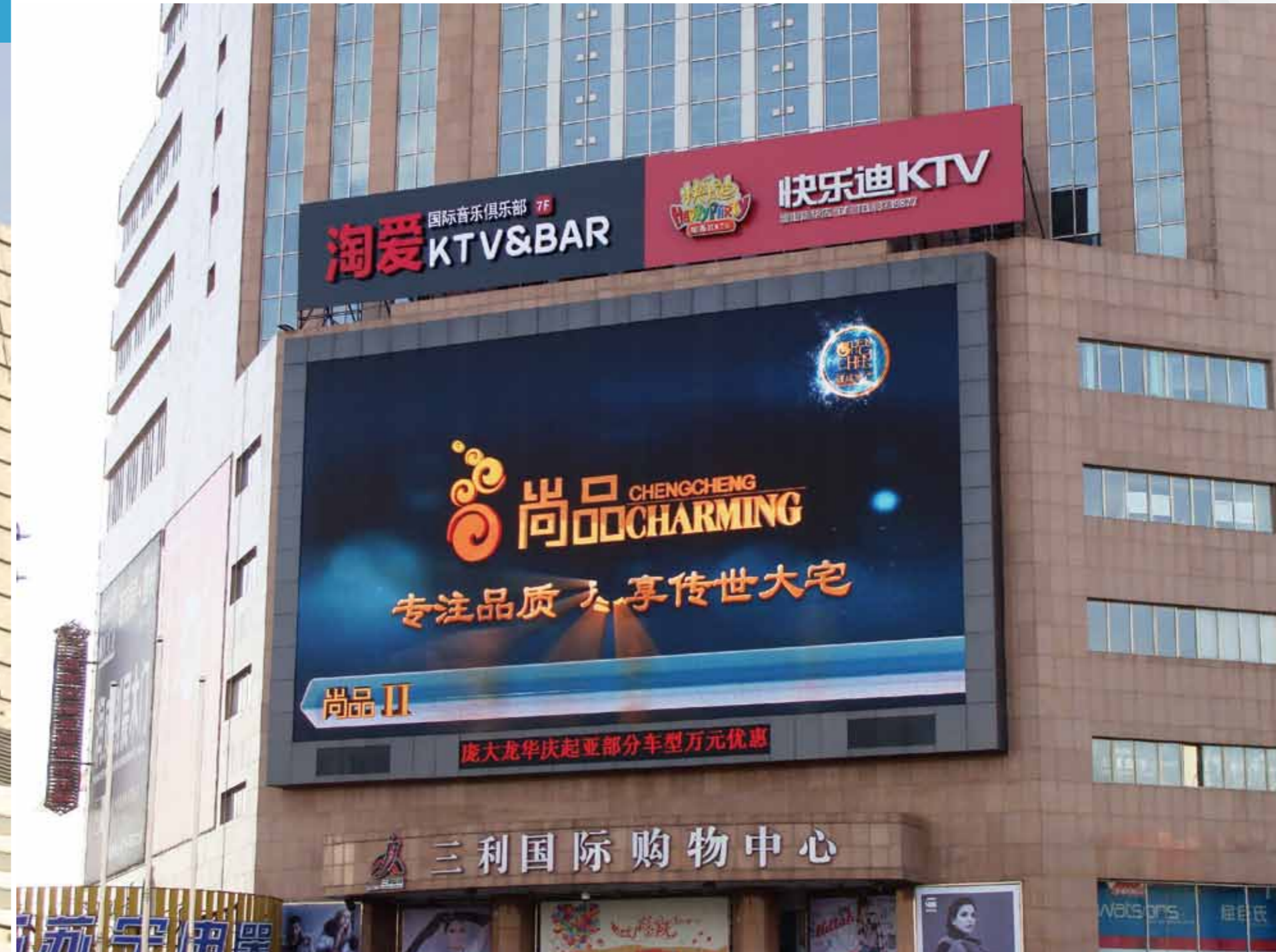
Tangshan Expo Building LV20A 351.4 m 2
